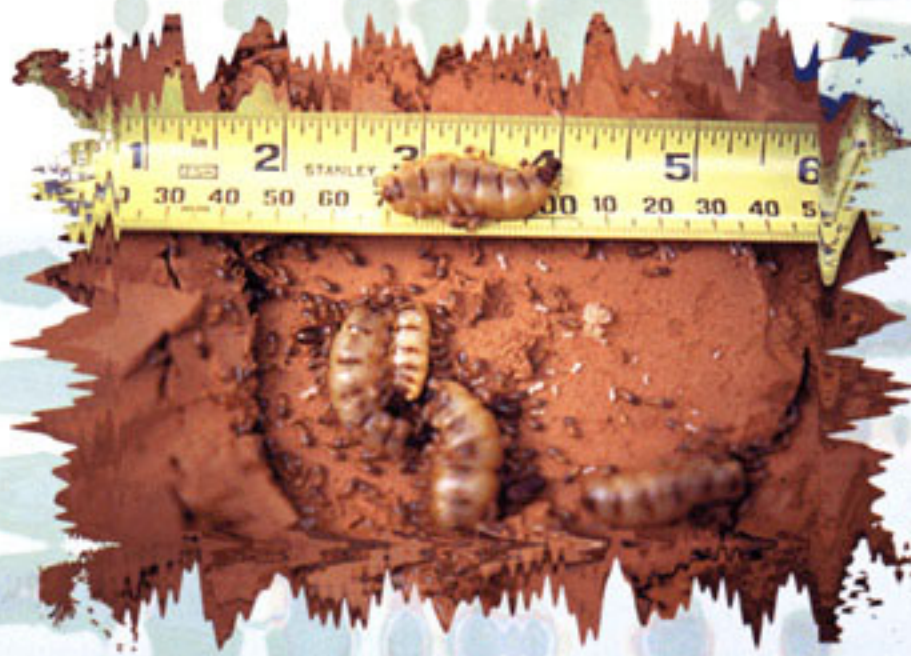
An established Subterranean Termite colony, nesting 5 queens, numerous kings, soldiers, workers and nymphs.
